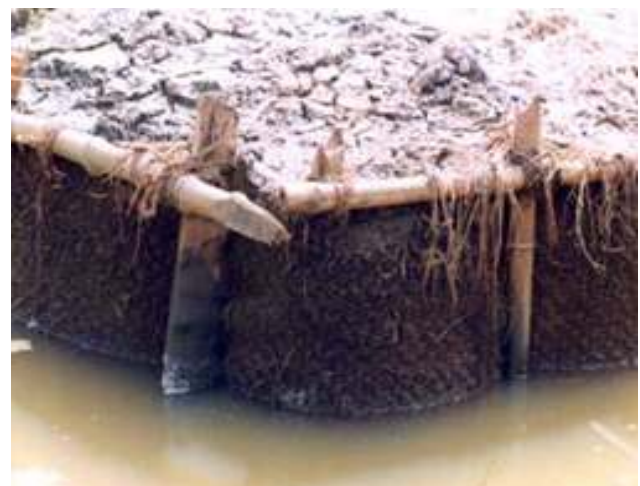
Figure 3: Close up view of applied coir geotextile on the stream bank
