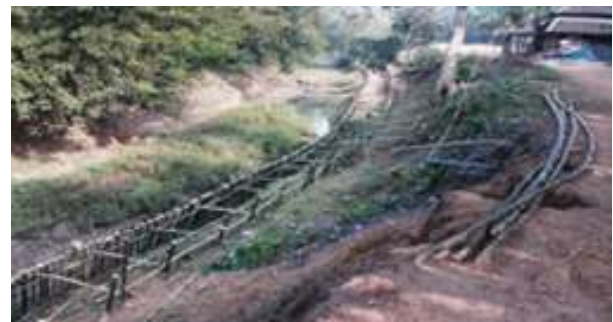
Figure 7: Aligning bamboo geogrids with bank geometry
