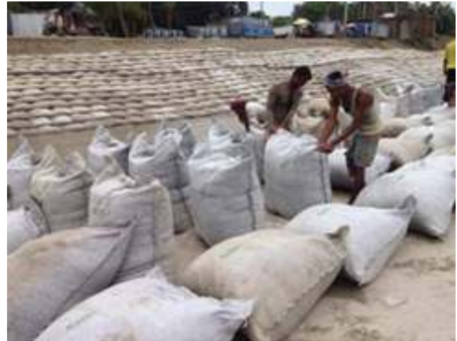
Figure 2: Counting and lengthwise placing of filled geobags
